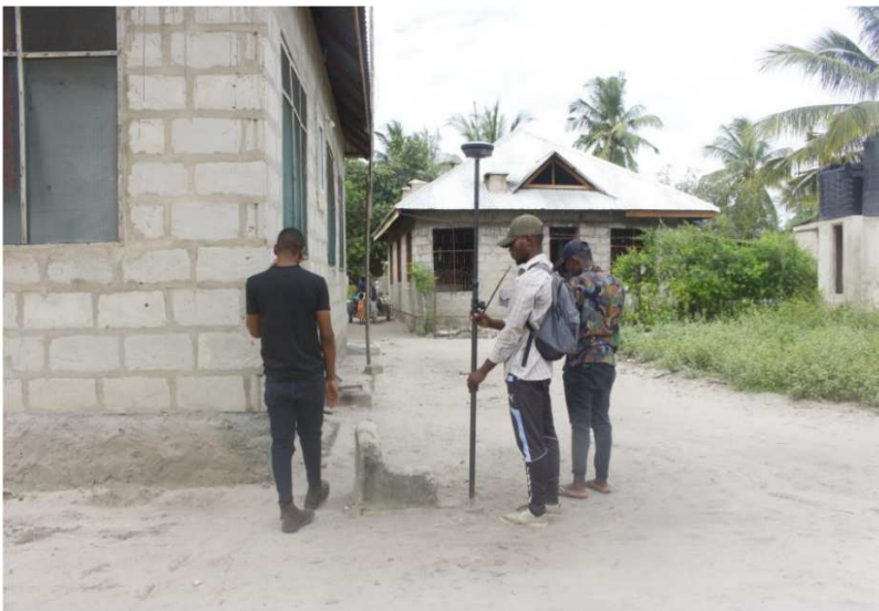
Fig 1: Land surveying for regularisation of Unplanned Settlements at Kivule in Dar es salaam
